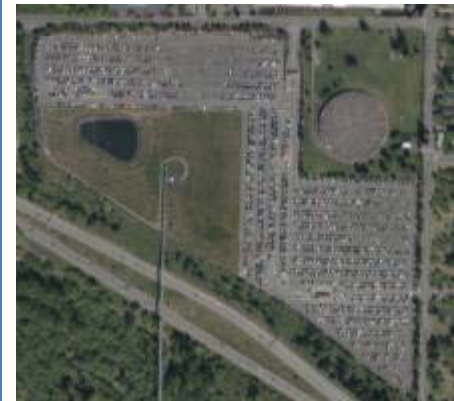
Existing NEPL Facility
