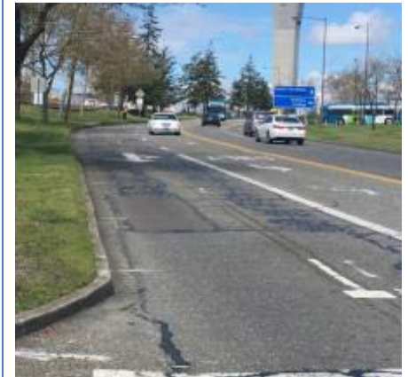
Existing Roadway Conditions
