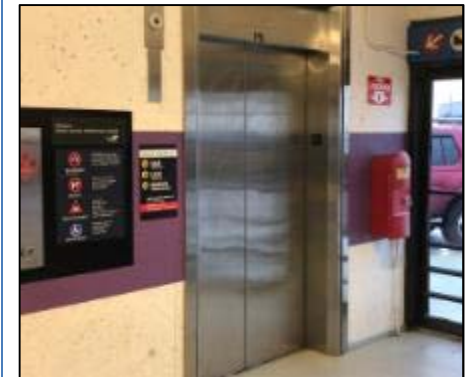
8 th Floor Elevator Lobby
